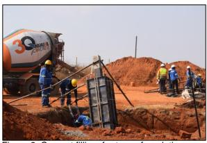
Figure 3: Cement filling for tower foundation
